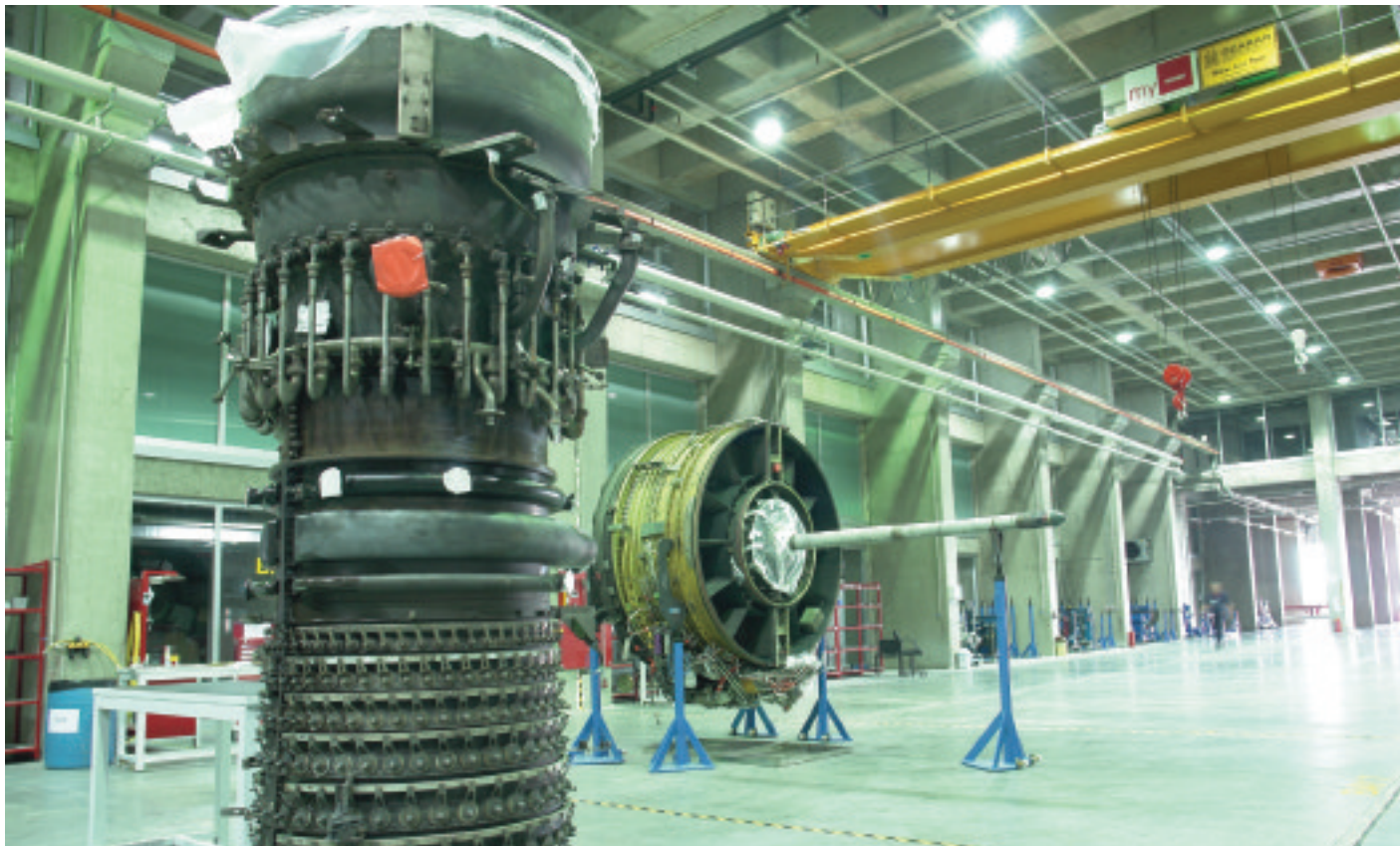
In the next five years, myTECHNIC aims to employ over 1,000 people, performing more than 300 C checks and around 50 engine overhauls annually.
